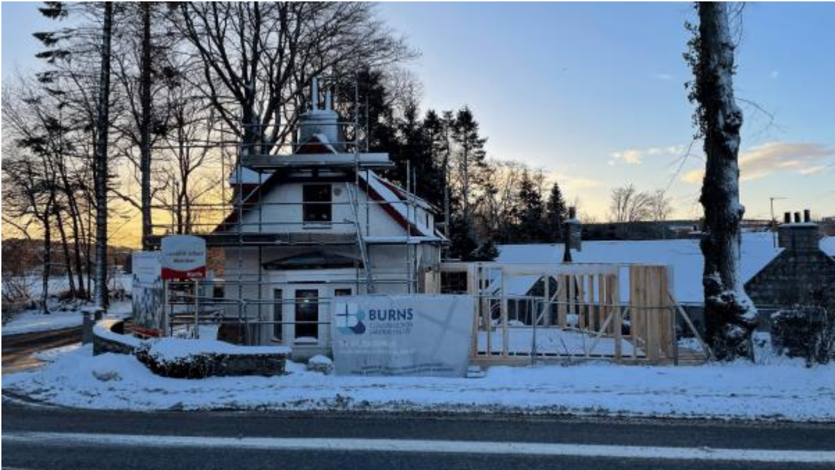
Construction in progress of Murtle Market
