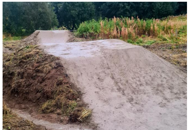
Jumps under construction
